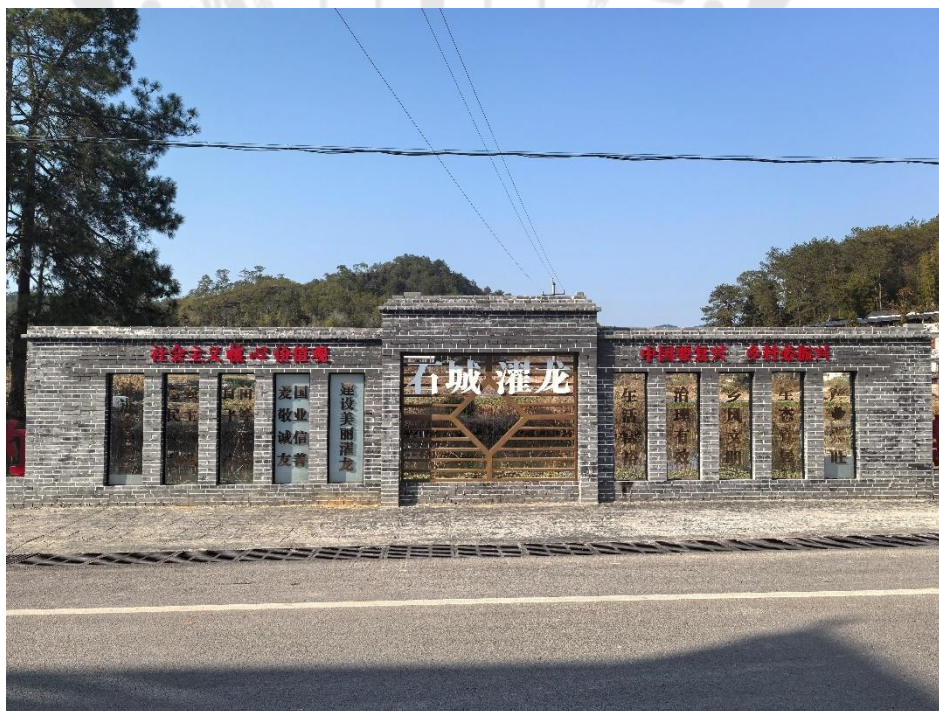
Figure 13 The Entrance to Zhuolong Village, Dayou Township
