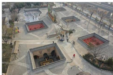
地坑院营造技艺 Construction techniques of underground pit courtyard
