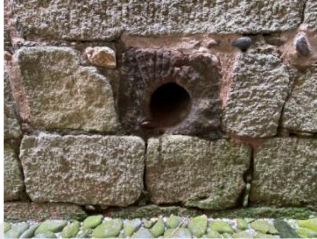
Figure 19 Sound transmission hole. Retrieved from https://zhuanlan.zhihu.com/p/355208201
