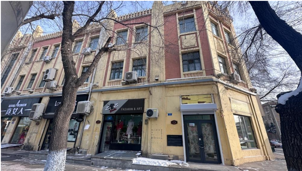
Figure 78 Harbin Railway Engineering Second Engineering Company
