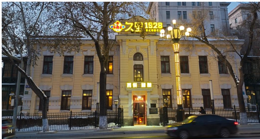
Figure 56 Residential Building No. 405 Fa Yuen Street
