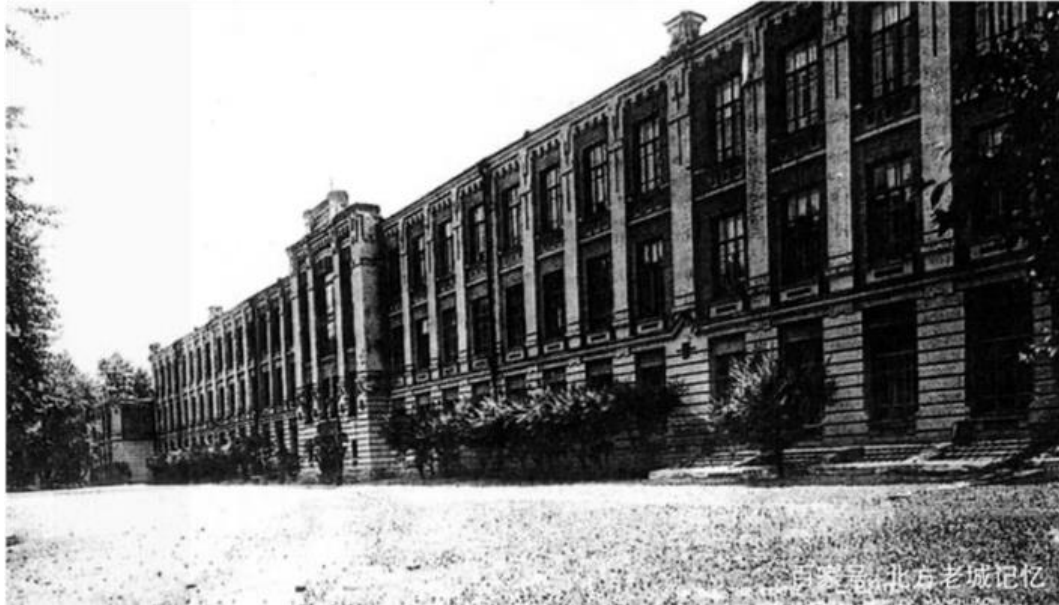
Figure 74 Air Force No. 1 Flight Academy Residential Building No. 2
