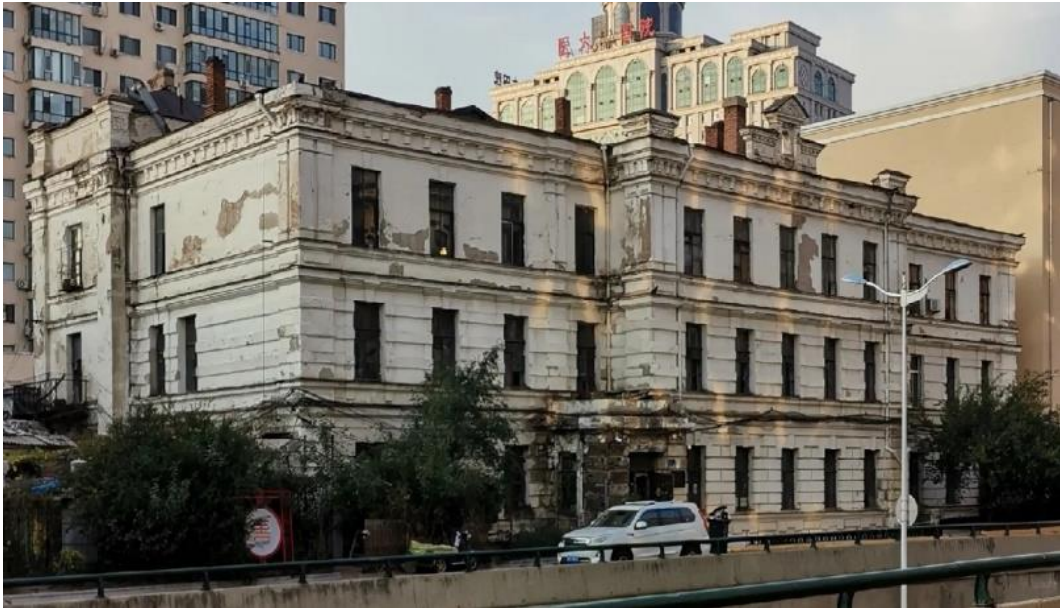
Figure 55 Building No. 93, Minyi Street
