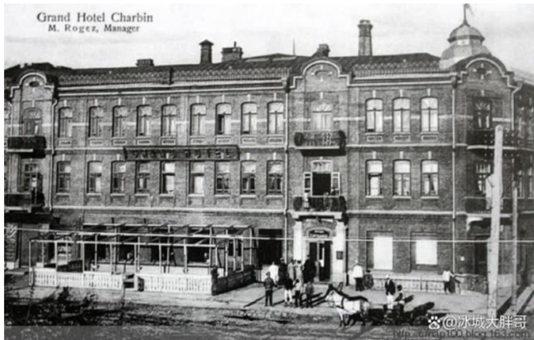
Figure 59 Harbin Grand Hotel (Former site)
