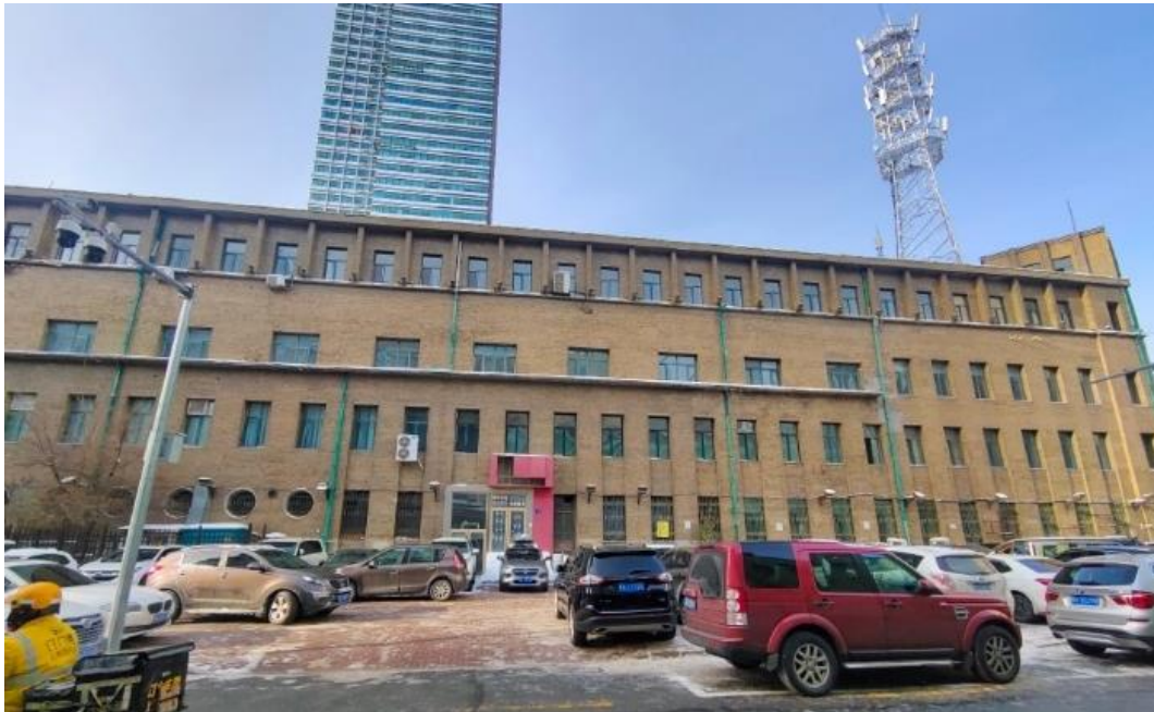
Figure 80 Harbin Telecommunications Bureau
