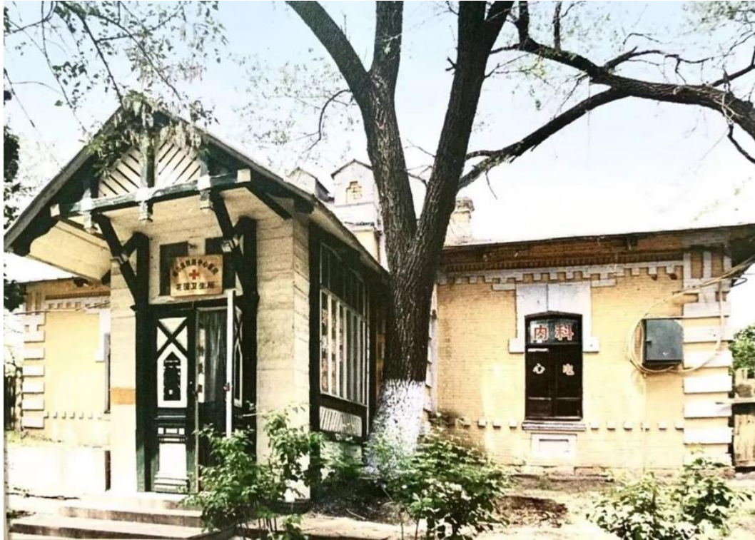
Figure 75 Harbin Railway Central Hospital Health Clinic
