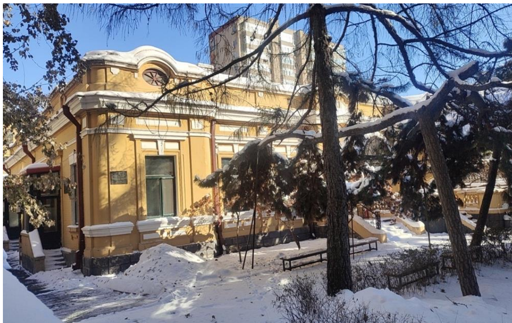
Figure 43 Residential Building No. 7, Liaoyang Street
