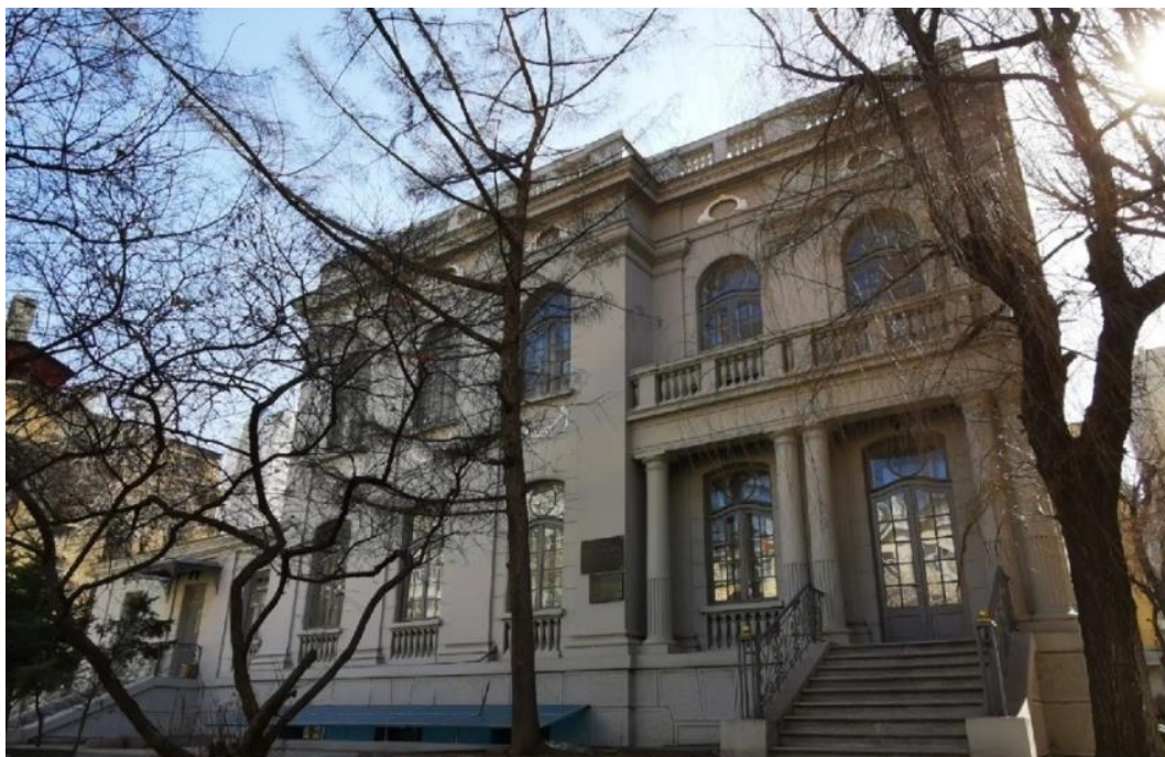
Figure 62 Residence No. 54 Jilin Street
