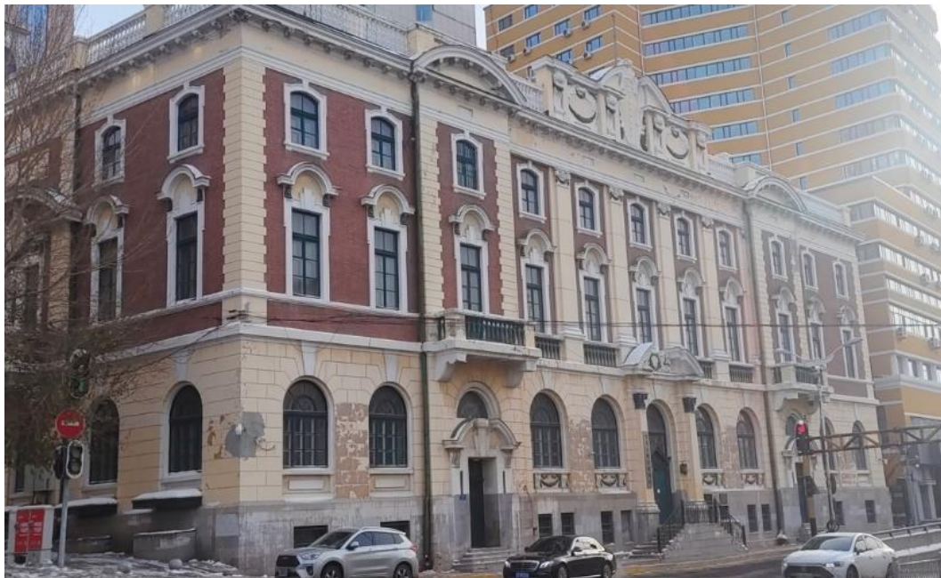
Figure 41 Heilongjiang Post and Telecommunications Administration Former Site Province
