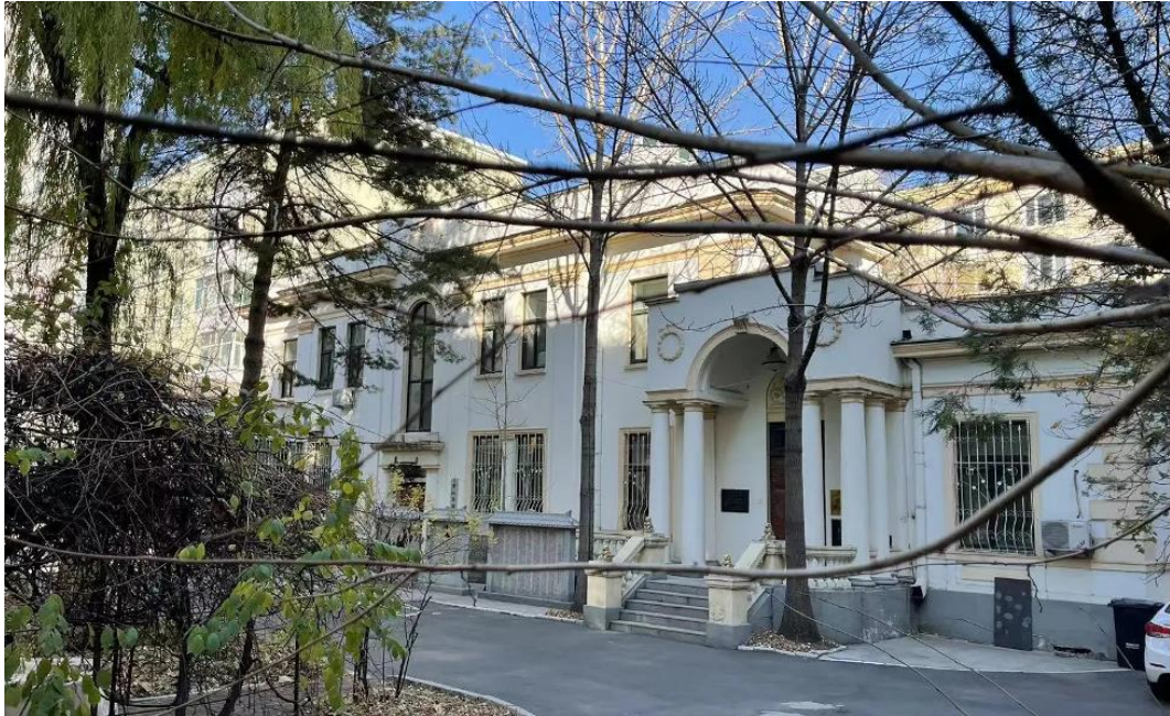
Figure 44 Residential Building No. 23 On Shan Street
