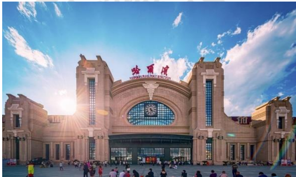
Figure 10 Harbin Railway Station
