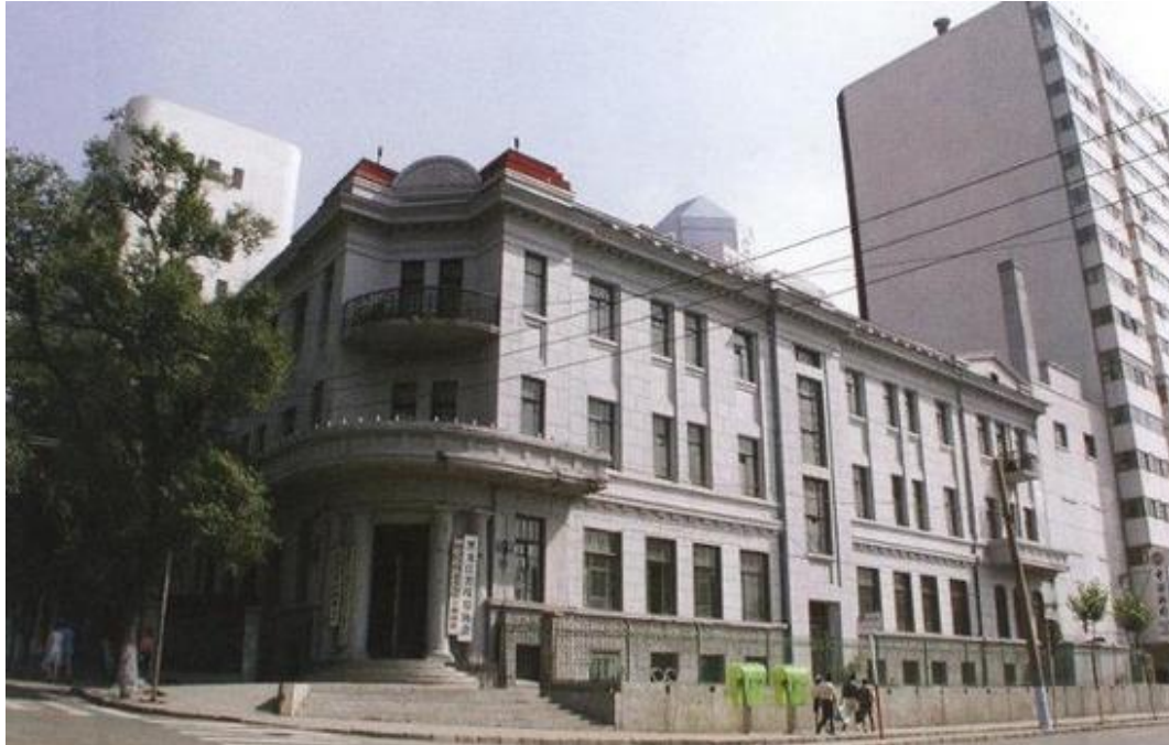
Figure 81 Former site of Beiman Special District High Court
