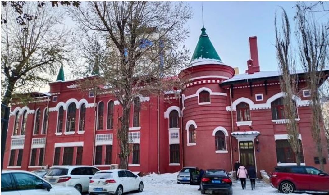
Figure 14 Central Telephone Bureau of the Middle East Railway
