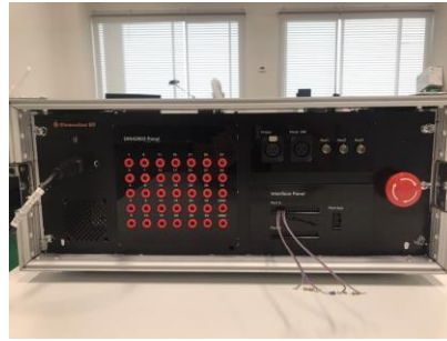
Figure 32 A 235-Ohm resistor connected to the machine.
